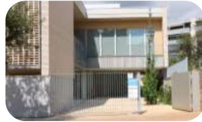
CAP Can Roca Terrassa
